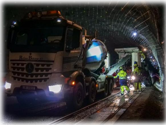
Foto: Ryfoss Betong AS - tunnelstøyping
